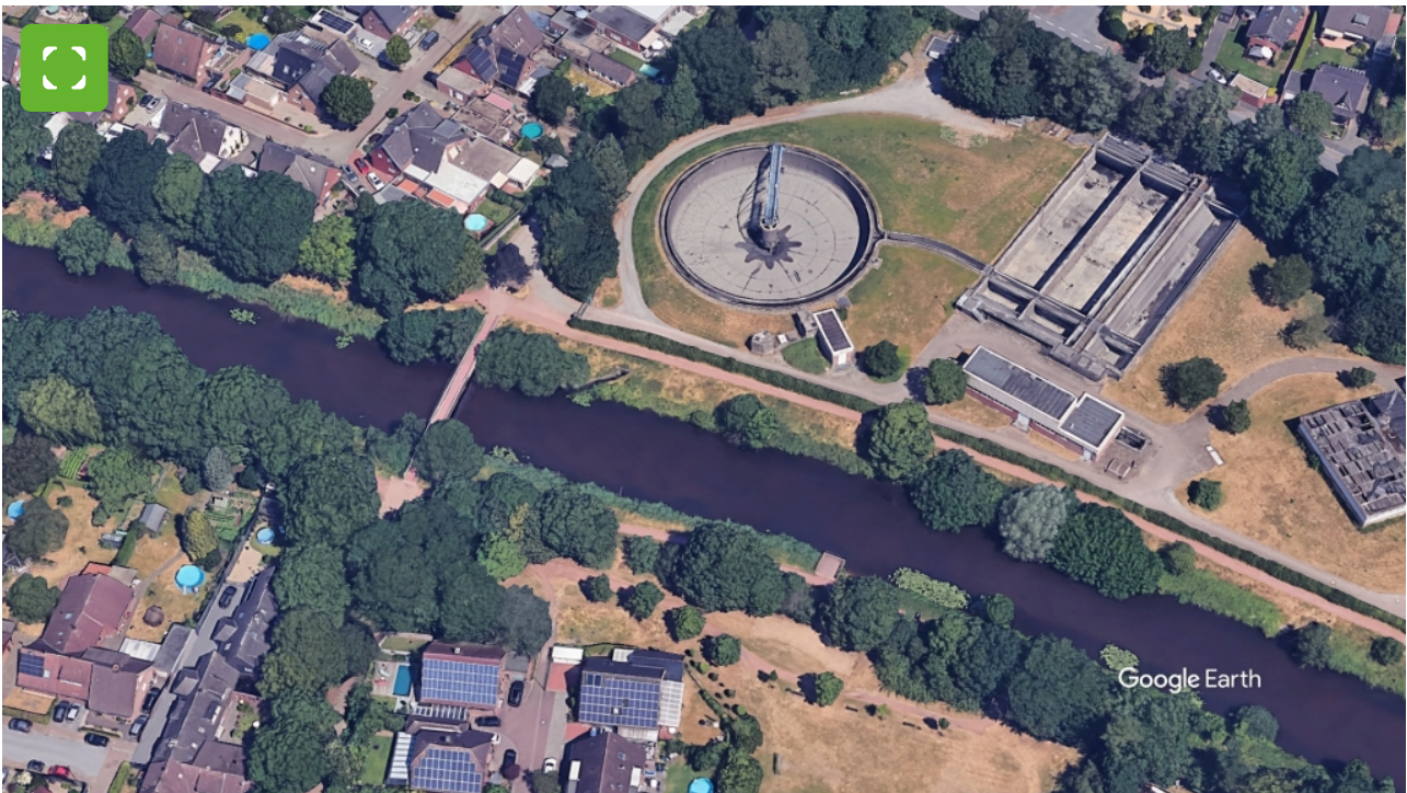
Aa bridge to be renovated © Google Earth
