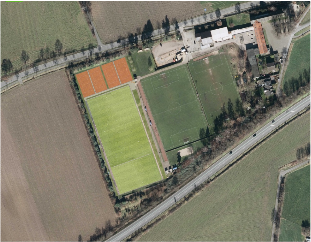
This is how the new sports facility of SC TuB Mussum with the new artificial turf pitches and tennis courts will soon look. The construction work has begun. © Stadt Bocholt
