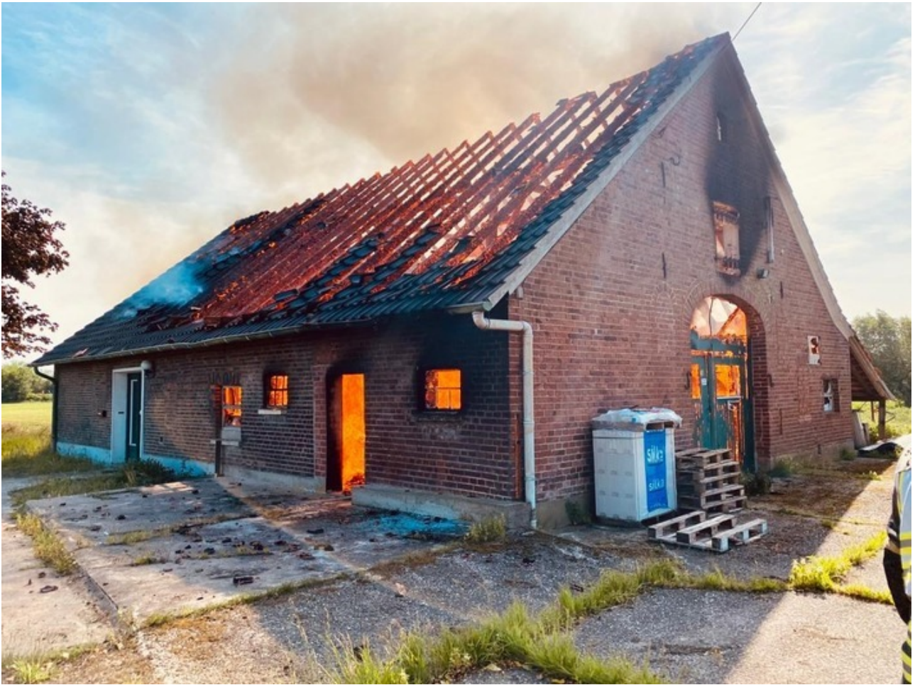
Building in full fire © Feuerwehr
