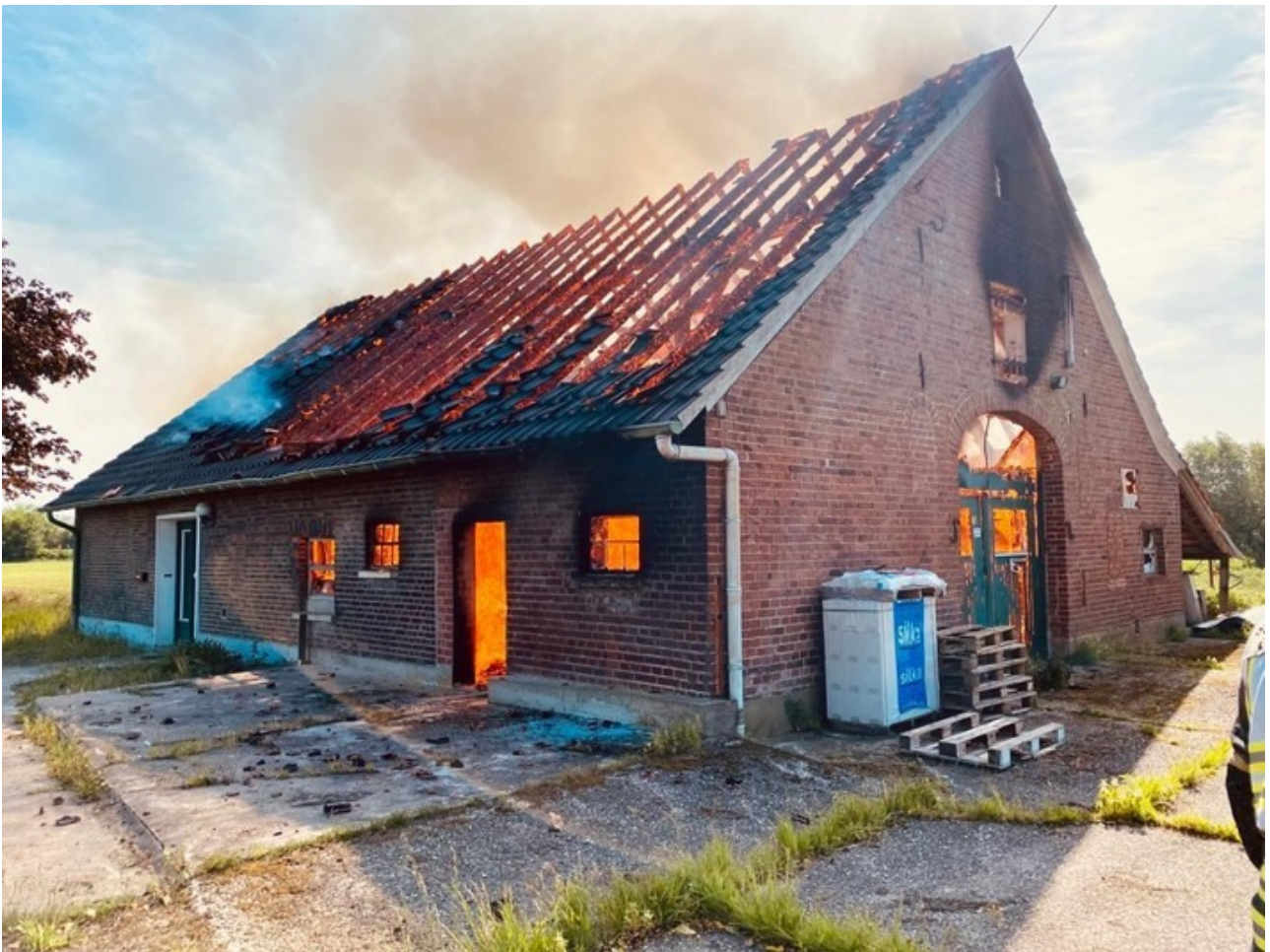
Building in full fire
