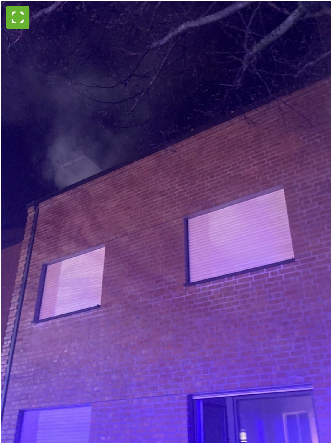
Picture during opening of roof window
