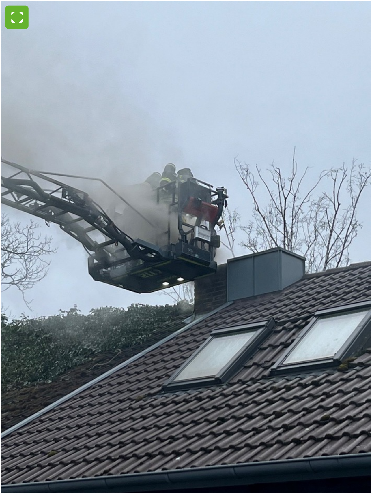
Burning chimney is swept from the turntable ladder basket. © Feuerwehr
