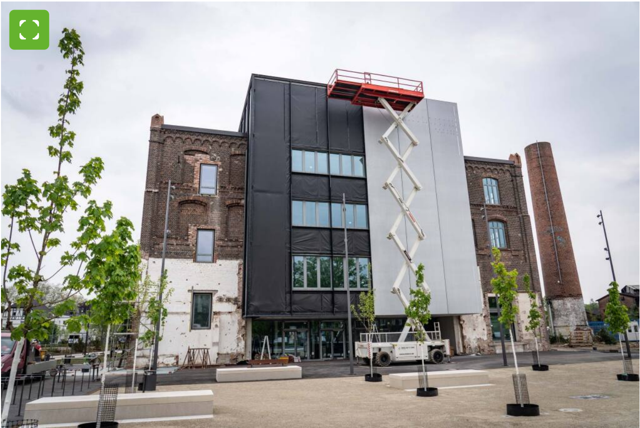
Workers use a cherry picker to attach the fabric panels to the building
