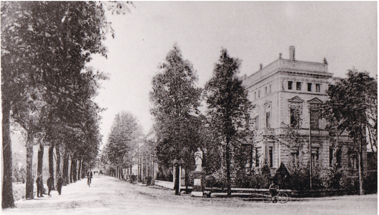
The former Villa Liebreich in Bocholt's Westend, shown here in 1905, was severely demolished inside by an SA squad on the night of the pogroms on 9/10 November 1938. Emilie Liebreich, badly beaten, had to be taken to hospital by "surreptitious means". © Stadtarchiv Bocholt
