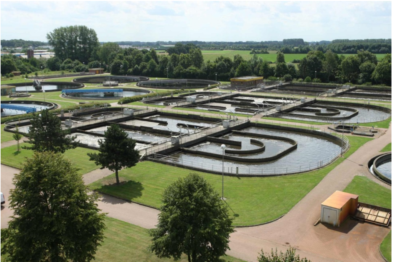
Sewage treatment plant in Bocholt (archive photo) © Stadt Bocholt
