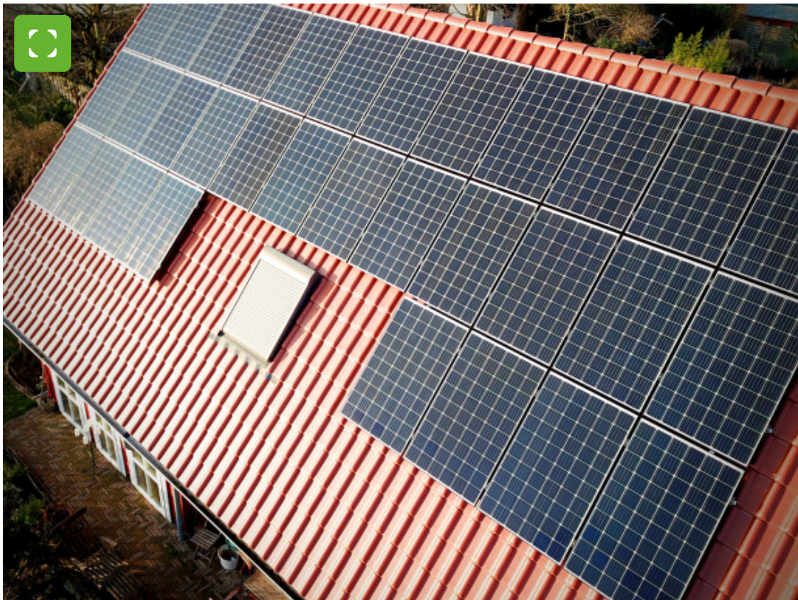
A solar system on the roof of the house
