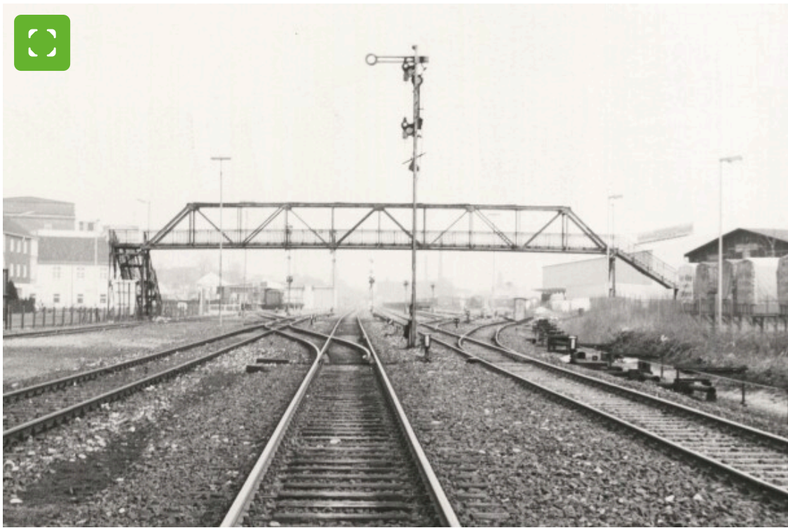
The railway bridge on Kaiser-Wilhelm-Straße
